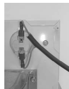
Figure 7-Lamp electrical connections
